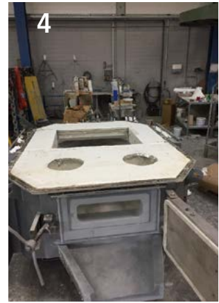
Figure 6: Installation of heating and roof blocks
