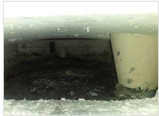
Figure 7: Condition of furnace after 3.5 years
