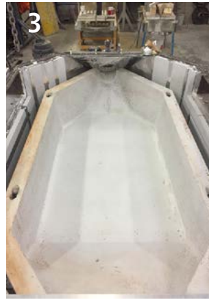
Figure 5: Installation of the liner
